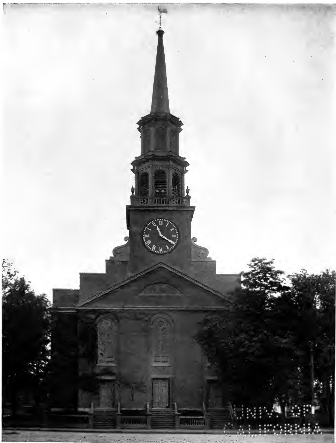
FIRST CONGREGATIONAL CHURCH, DOVER, NEW HAMPSHIRE
